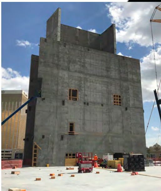
Core 3 has been topped out.
